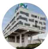
Hospital South Gai Gon VIETNAM
